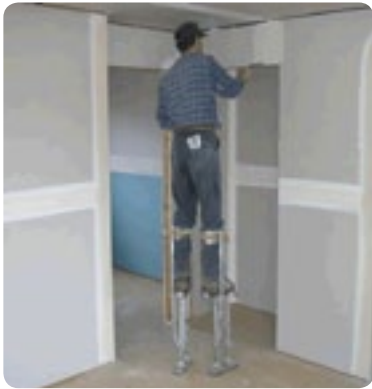
Figure 26: A plasterer uses stilts to comfortably reach above door frames.
